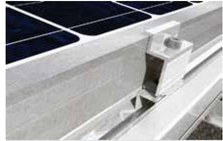
Detail: fastening of PV module
